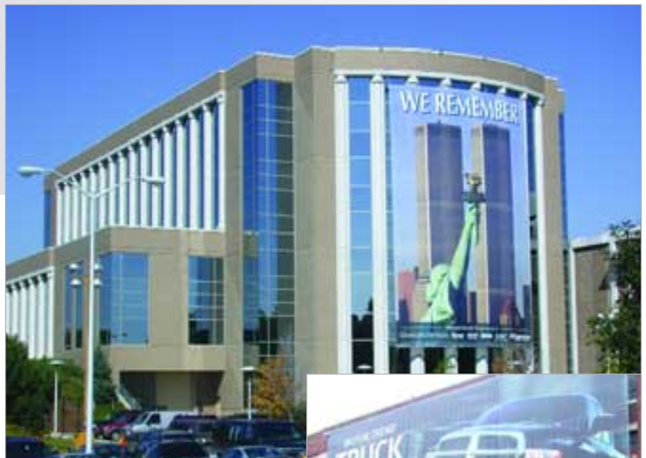
This 40' x 62' banner was created to honor the anniversary of the 9/11 tragedy. Although the face of the building is curved, Northstar's custom mounting hardware allowed the banner to follow the curved surface without it actually touching the building.
